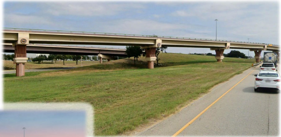
Existing view at Texas Ave. overpass
